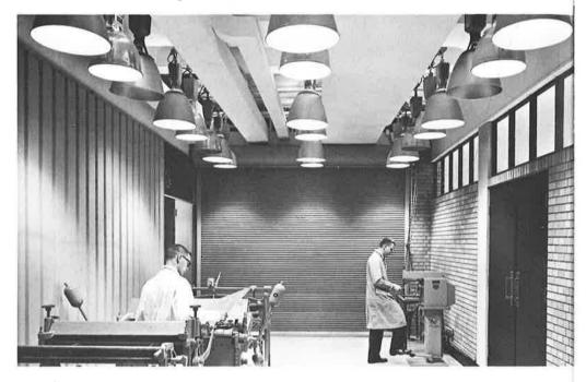
De Luxe White Mercury and colorimproved mercury lamps are operated in fixtures providing 10 per cent and 15 per cent upward light component. Low-brightness reflector interiors show that units can be mounted in lowceiling areas without visual discomfort to occupants. Of course, reflectors have to be deep enough to prevent direct glare from the light sources.
