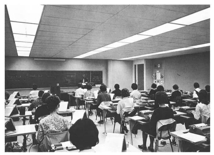
This is an interior classroom. Air is circulated through the lighting fixtures, and both body and lighting heat
