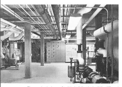
The mechanical area for this building looks little different from comparable ones in office buildings. The suspended fixtures are well shielded, and placed where the light is needed most. Above the control board is a single-lamp unit that directs light evenly down and across the board so that all of the control devices and meters can be read easily.
