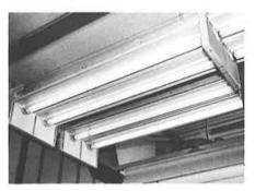
A mirror at the top of the movable partition doubles, in effect, the lighting systems. Actually, there are only three fixtures in this one. Each contains two, 48-inch high-output lamps. Fixtures have movable side panels and center V section so that shielding angles from 0° to 45° can be demonstrated (see other pictures). Also, as shielding angle is increased, upward light increases. The maximum amount is 25 per cent.
