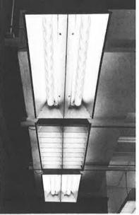
Six fixtures, each containing four-foot Power Groove lamps, can be rotated to demonstrate crosswise and lengthwise shielding. One side (interior) of each unit is white enamel. The other side is anodized aluminum. The sides reflected in the mirror also help to show the effect of brightness control of a lighting system in a room. Upward light component is variable (depending upon the fixture), and it is pointed out that this component should be about 25 per cent.
